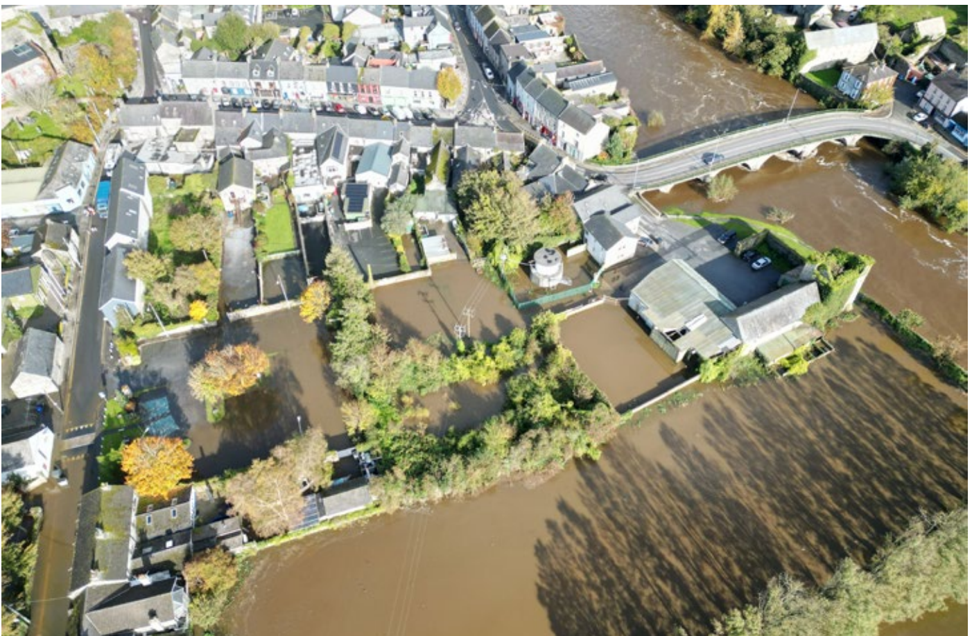
Flooding in Thomastown from Storm Babet in 2023
