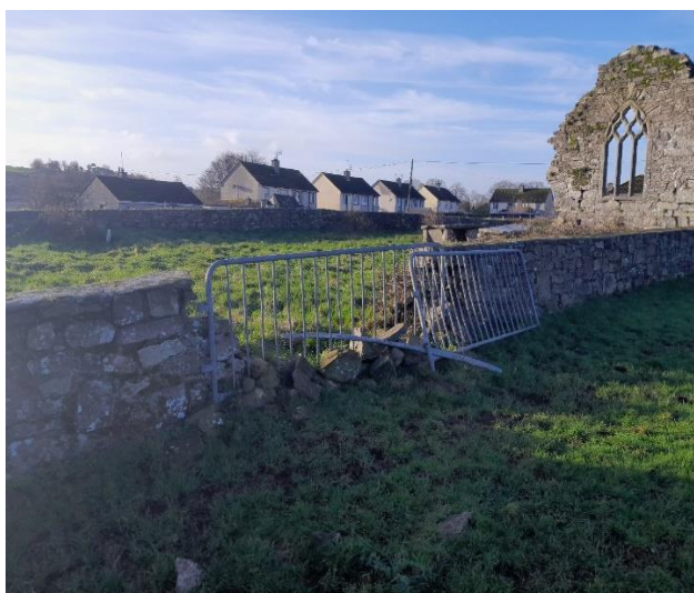
The Thomple in Thomastown where conservation works will be commencing soon
