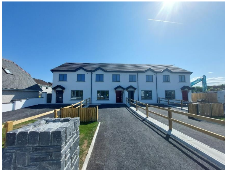
The above photo is 4 units now completed at Breagh Terrace, Main St, Piltown
