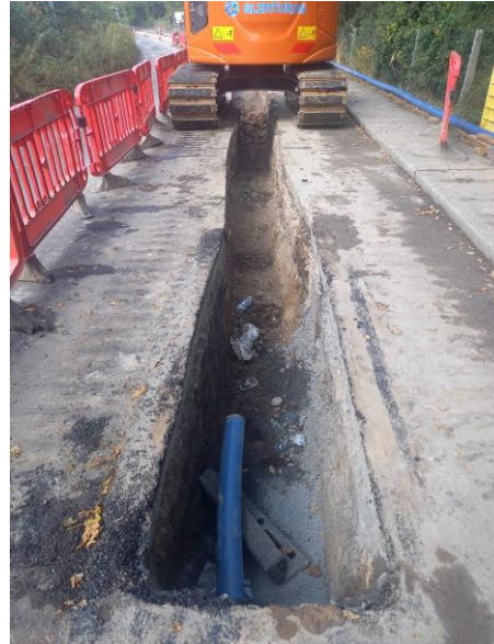
Construction of new HDPE water-main at Slieverue Village
