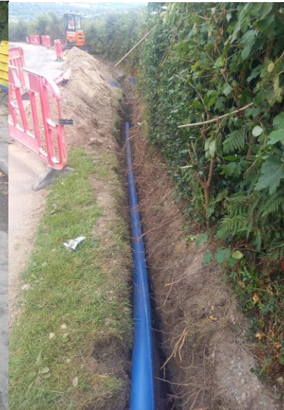
Construction of new HDPE water-main at Carrickmourne, Thomastown
