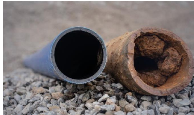
Typical existing Cast Iron Main condition versus new HDPE Main
