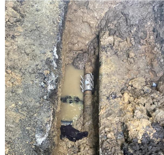
Leak Repair in Annamult, Bennettsbridge
