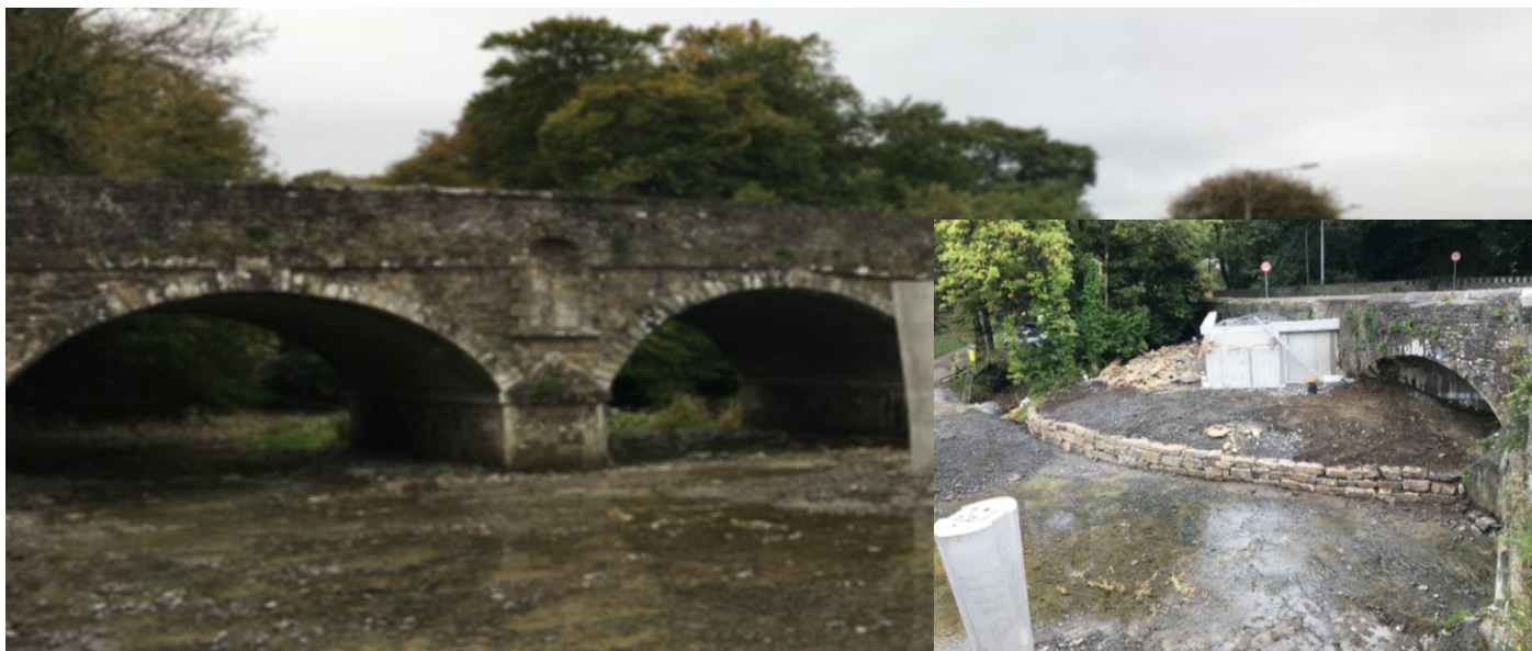
Central Pier Completed and river reinstated
