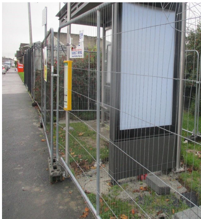
Bus Shelter Provision at Larchfield - SHELTER INSTALLED
