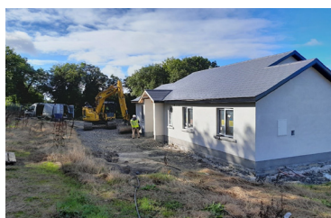
Construction of rural houses at Shanganny, Jenkinstown
