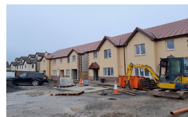
Construction at Limegrove, Belmont. 3 bed houses.
