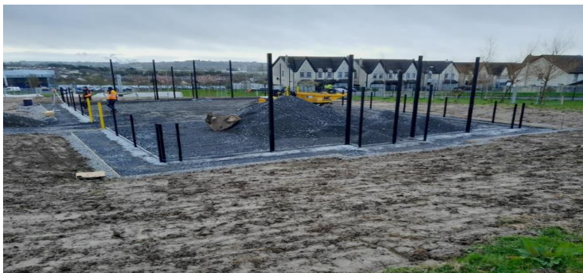
Progress of new MUGA in Ferrybank Neighbourhood Park
