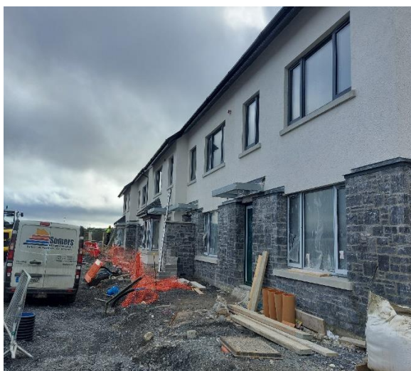
Legan Grange, Thomastown (25 units due in Q2 2023)
