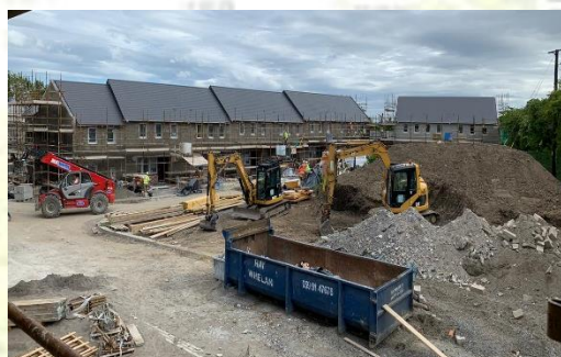
Glebeside, Donaguile, Castlecomer - 33 units under construction
