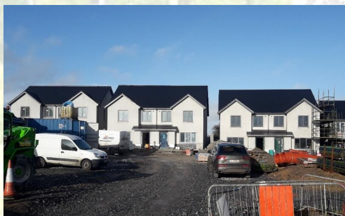
Breagh Place, Piltown – 17 units under construction
