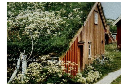
Fig.2.04.3 Green roof, Norwegian house
