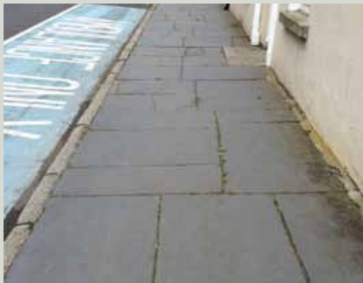
Limestone flags in Monasterevin, County Kildare
