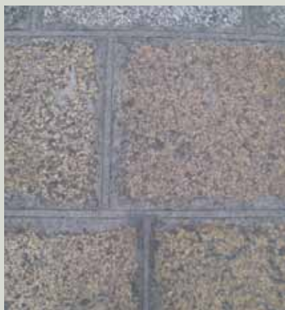
Inappropriate pointing: these four examples show crudely applied pointing using methods and materials which are inappropriate for historic paving. The use of cement-based mortars will damage the stone in the long term whilst the damage to the visual appearance of the paving is immediate.
