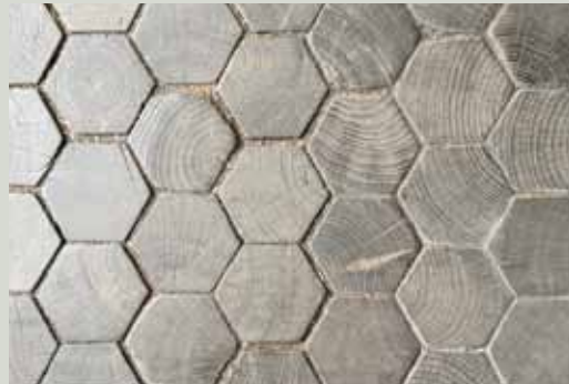
Some rare surviving hexagonal timber setts in the archway leading to Front Square in Trinity College Dublin
