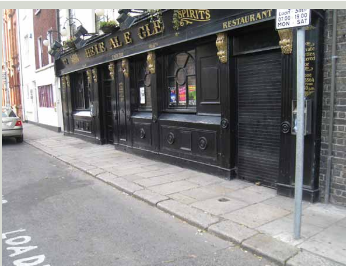
Granite flags and kerbs retained outside a public house on Chancery Place, Dublin
