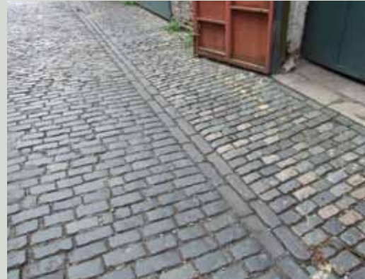
Gutter detail in North Lotts, Dublin
