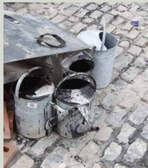
Cans for tar grouting
