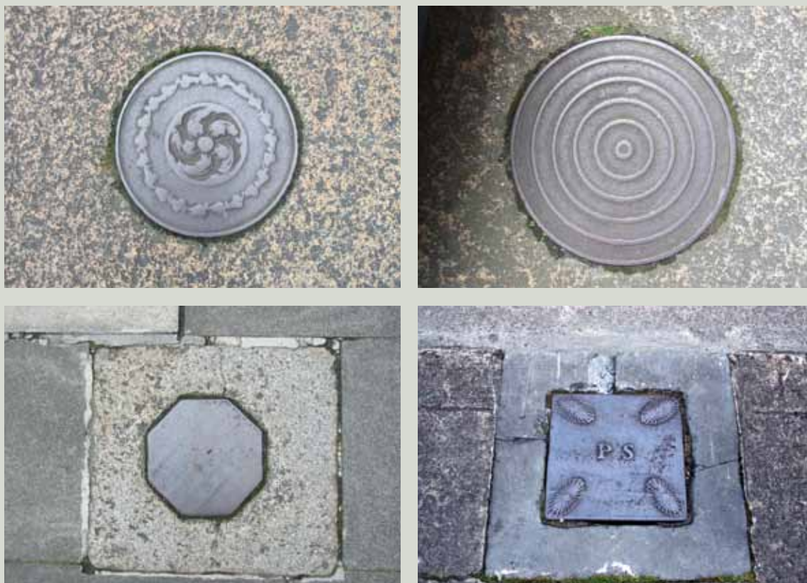
Coalhole covers: Fitzwilliam Square, Dublin and Pery Square, Limerick. A meeting of the Dublin Paving Board in 1774 required that: 'all the stoppers of Coal Vaults, in the Foot Paths, or Carriageways, be made of cast metal not under one inch thick'
