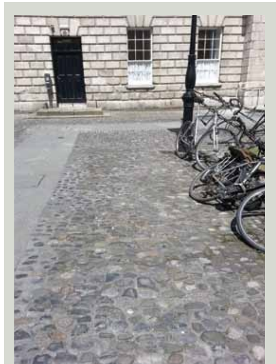
Cobblestone paving in Trinity College, Dublin. Although this paving has been re-laid several times, many of the cobblestones may date from the original mid-eighteenth century creation of Front, or Parliament, Square
