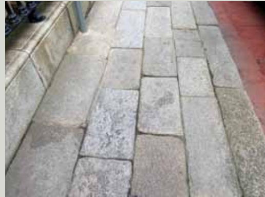
Granite flagged pavements are found in several towns along the east coast, including this example at Commercial Quay, Wexford
