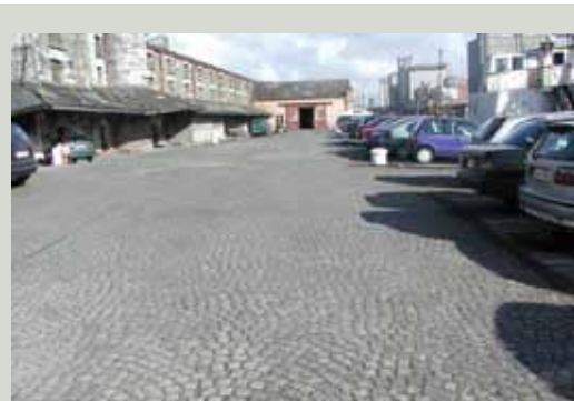
Stone setts dating from c.1815 adjacent to a bonded warehouse complex in Cork City. The fan-shaped pattern used in the layout of the setts is unusual in Ireland and may point to the involvement of continental workers
