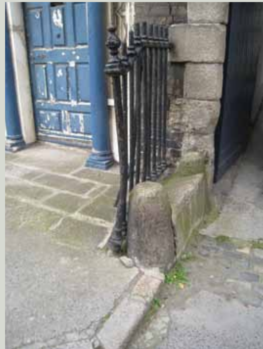
Stone bollards, or jostle stones, were used to protect buildings from damage from vehicles
