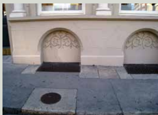
Pavement features such as pavement lights or cellar access hatches were provided with stone surrounds. Where only a remnant of the stonework survives, it should be an objective of any repaving works to replace the missing stones in order to re-establish the complete surround
