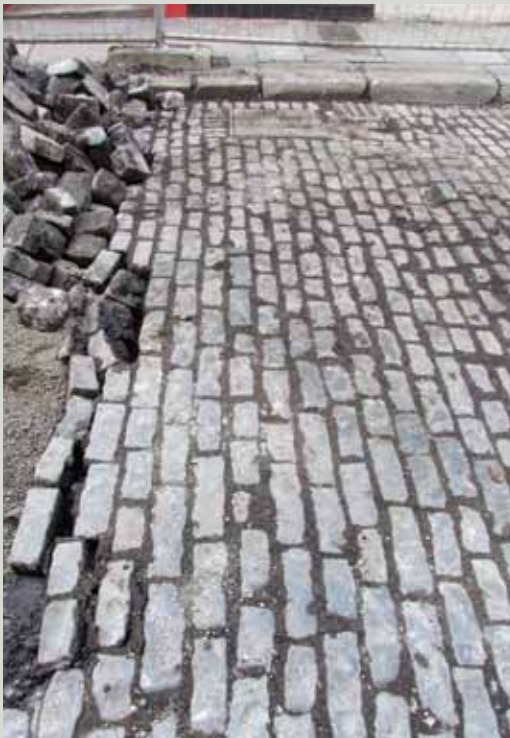
Setts laid in tar being taken up prior to being re-laid
