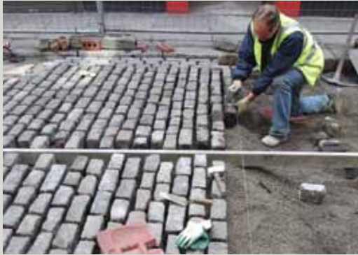
Sett-laying in rigid construction without contact between setts. Note inconsistent joint width which is a result of the setts not having been sorted according to size.
