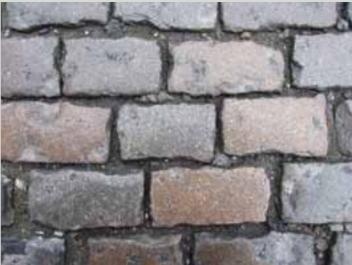
Green diorite setts in North Lotts and granite setts at Haymarket, both in Dublin. The consistent size of the setts and the narrow joints are characteristic of the original craftsmanship that went into laying these pavements
