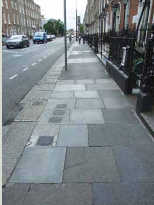
Access covers installed along a highly significant Georgian street have created a patchwork of different materials and flagstone sizes which disrupt the appearance of the Neo-classical street
