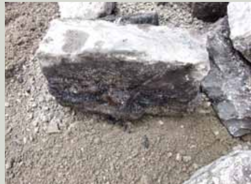
Cold tar jointing material on a salvaged sett is disfiguring and difficult to remove from the historic stonework
