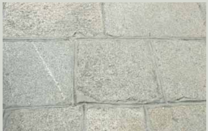
Inappropriate pointing: these four examples show crudely applied pointing using methods and materials which are inappropriate for historic paving. The use of cement-based mortars will damage the stone in the long term whilst the damage to the visual appearance of the paving is immediate.
