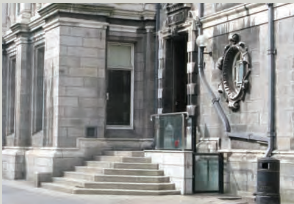
Mechanically operated short-rise lift systems using high quality materials can be sensitively integrated if well designed
