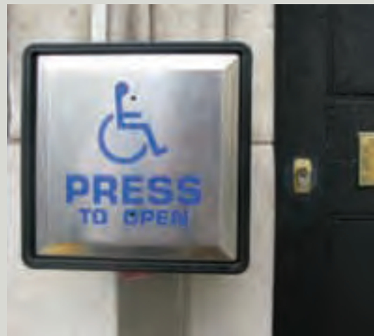
Power-assisted doors may be essential especially when the door controls are inaccessible or the door closers too strong or where door handles are too high
